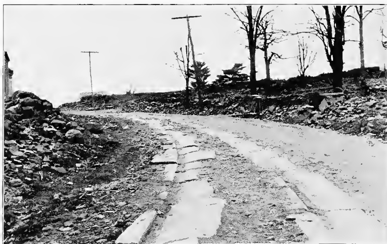
ROAD WEST FROM KINGSTON, ULSTER CO., N. Y., 1902. Built by Turnpike Company in 1862. STONE WHEEL-TRACKS.
